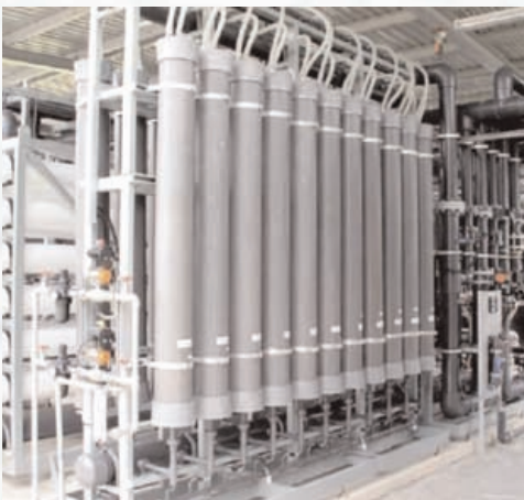
Jurong Industrial Water – 2,000 m 3 /day reuse for high grade industrial and DI water
